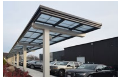
Bernard A. Greenheck Education Center, Schofield, WI, Ellis Stone Construction
