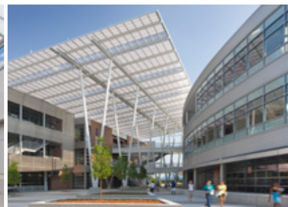
▲ Project: UNF Student Center ID: 24863 Location: Jacksonville, FL Architect: Rink Design Partnership
