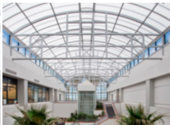
▲ Project: Hologic, Inc. ID: 34563 Location: San Diego, CA Architect: Smith Group Consulting
